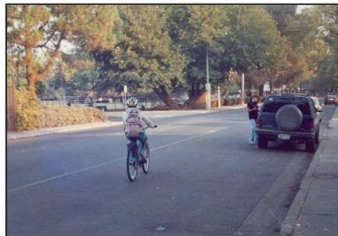
Wide Paved Shoulder Source: www.pedbikeimages.org / Laura Sandt
