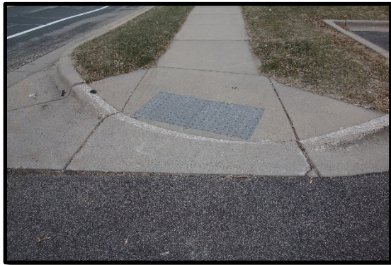
Curb and gutter at pedestrian ramp shaved
