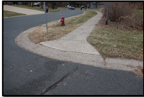
Concrete walk edge shaved
