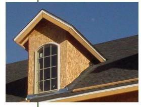
The intersection between the roof and the wall of this dormer should have a good water management strategy.
