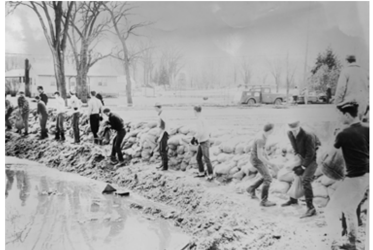
The community, including many teenagers, came together to help out with sandbagging after the flood in 1965.
